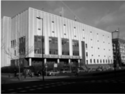
The converted cocoa warehouse in Amsterdam, home to NEHA since 1989
